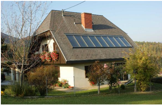
Fig. 2. Example of a one family house in Austria with a 18m 2 collector on the roof.
