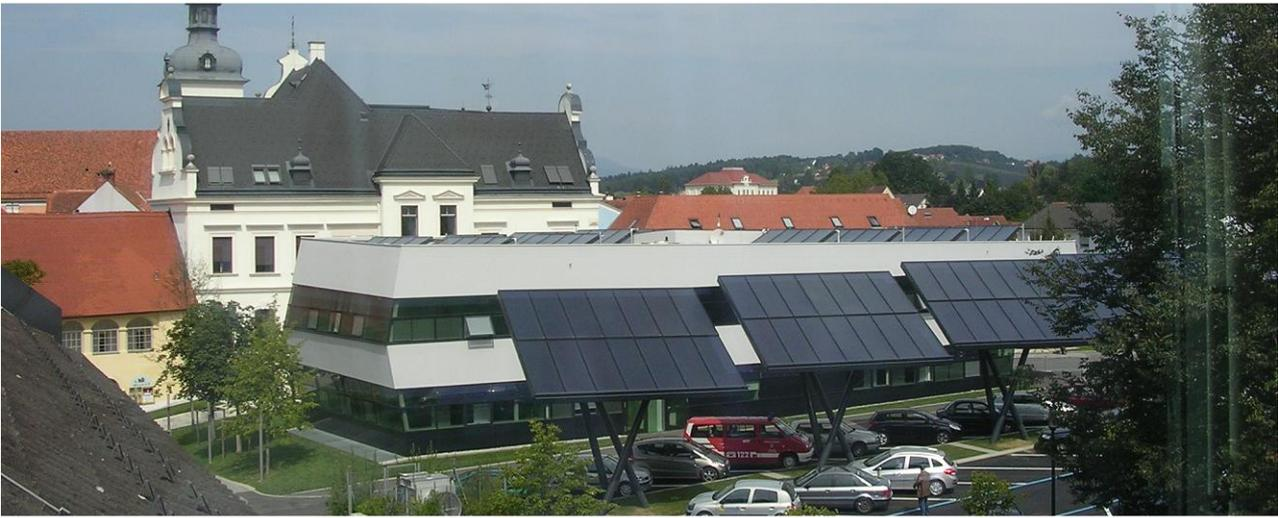
**Fig. 3. The entire project with solar thermal collectors mounted on „solar trees“ in front of the service center facing east and solar thermal collectors mounted on the roof facing west**
