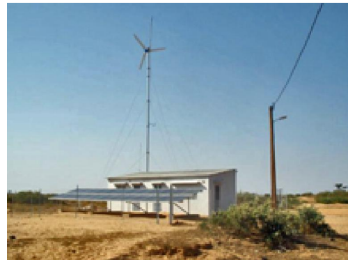
Fig. 2. Solar wind Diesel hybrid power system for small village
