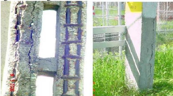
**Fig. 20. Steel concrete support elements (operating in high level electromagnetic field) degradations [22]**
