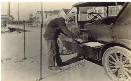
**Fig. 15. Mobile auto-laboratory designed for stray currents monitoring (Los Angeles 1910).**
