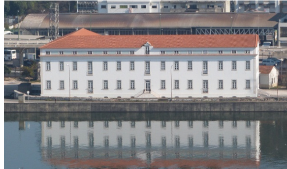
Fig. 1 - Pilot Building in Coimbra
