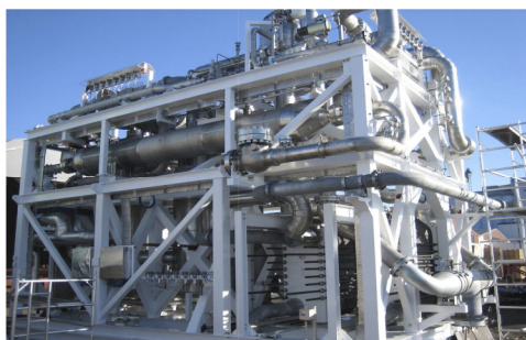
Fig. 9. Regasification trains
