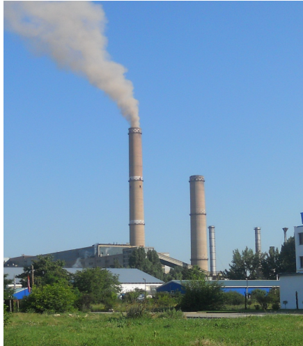
Fig.1. Cogeneration Thermal Power Plant of Oradea
