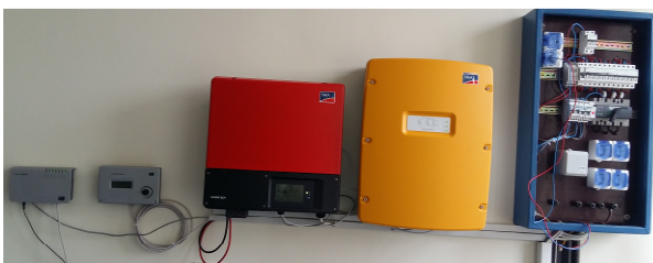
Fig. 2. Sunny Boy and Sunny Island inverters
