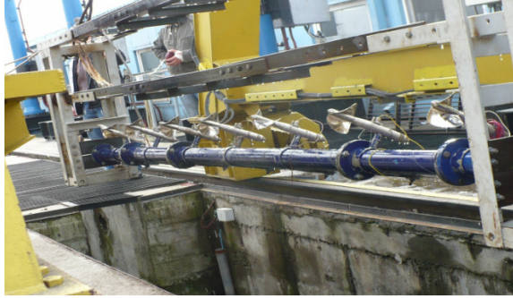
Fig.3 Current meter frame ready to be installed in the cofferdam recesses
